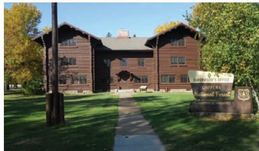
Old & new forest service supervisors office
