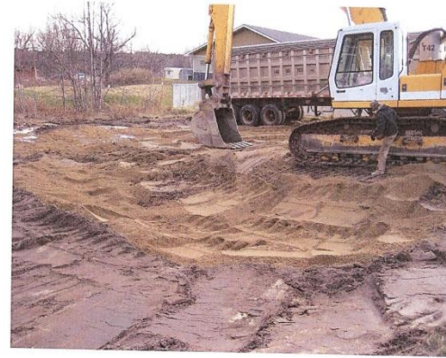
Photo 17 - Another view of the partially completed backfilling activities.
