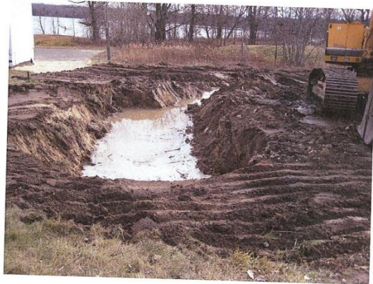
Photo 14 - Another view of the completed soil excavation and demolition activities.
