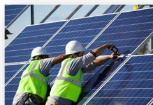
Solar PV installation
